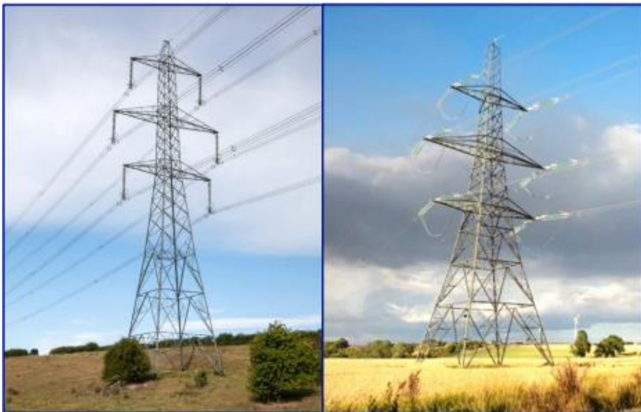
Image 4.2 Suspension tower (left) and Angle tower (right)
